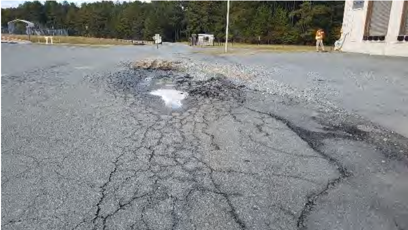
Figure 37 Jefferson Labs Road Infrastructure
