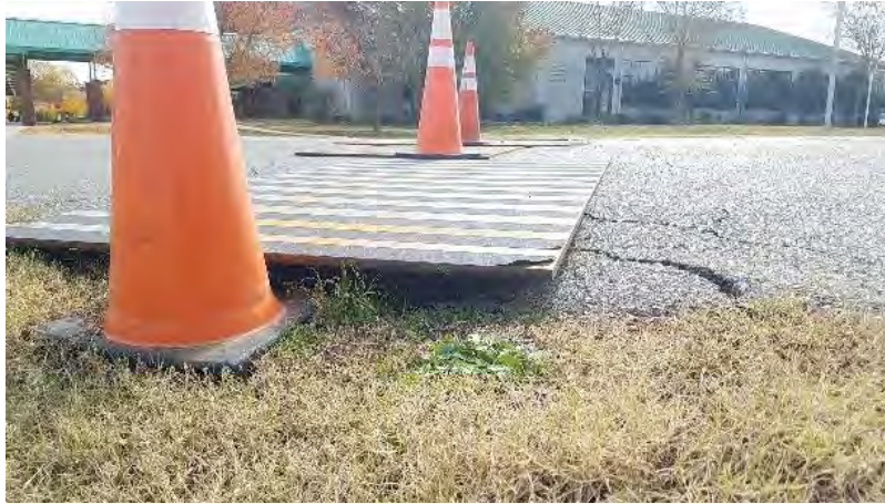
Figure 38 Jefferson Labs Road Infrastructure
