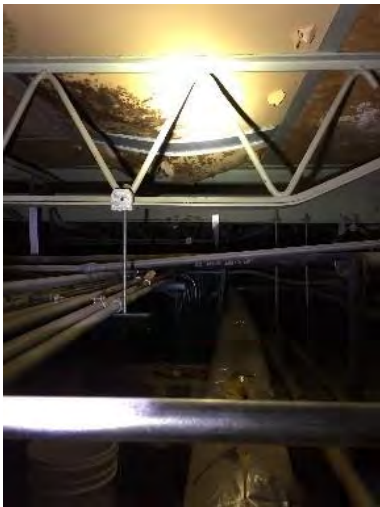
Figure 35 Jefferson Labs Roof Deck
