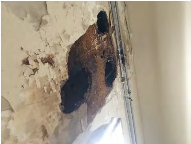
Figure 34 Jefferson Labs Roof Deck
